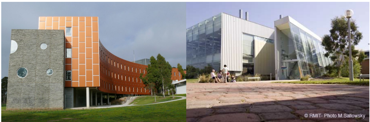
Figure 1: City campus (top); Bundoora campus (bottom left); Brunswick campus (bottom right)
